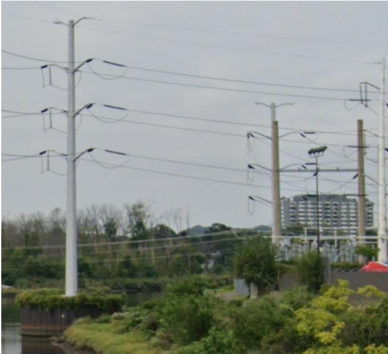
Figure A-5 Transmission power pole located near Arlington WPCP
